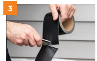
3 CUT TAPE TO THE DESIRED LENGTH
