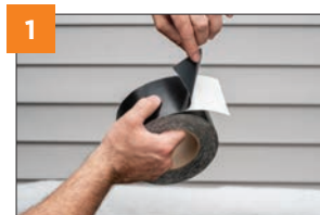
1 PEEL BACK THE RELEASE PAPER
