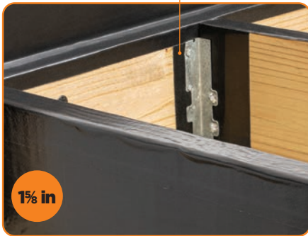
A BETWEEN JOIST HANGERS AND LEDGER BOARD
